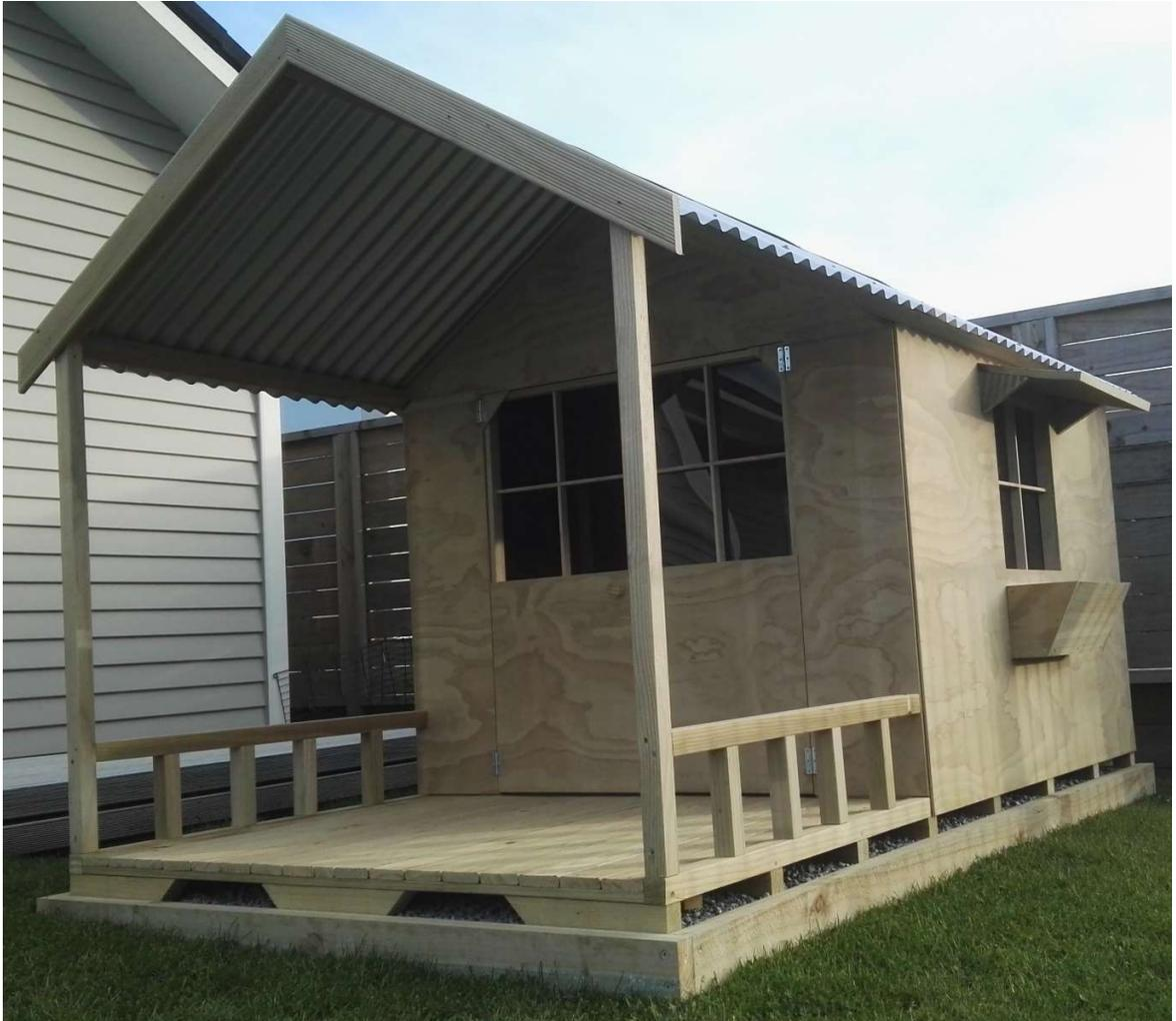
The picture shows the Wendy House sitting on top of the constructed platform. The pads of the floor can be seen sitting just inside the perimeter of the platform.
