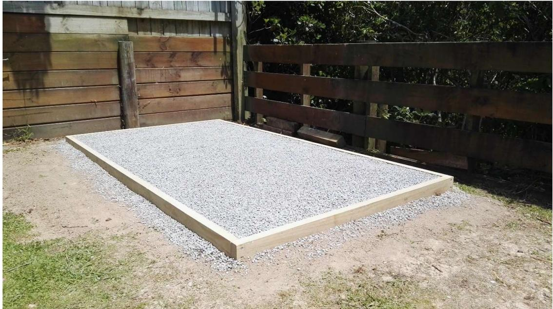
7. Place the floor panel of the Wendy House on top of the pea-metal inside the wooden surround. Titivate where necessary to provide an even support to all 24 pads on the base of the floor panel. Refer to pictures. If done correctly, the floor should feel solid to walk around on.
