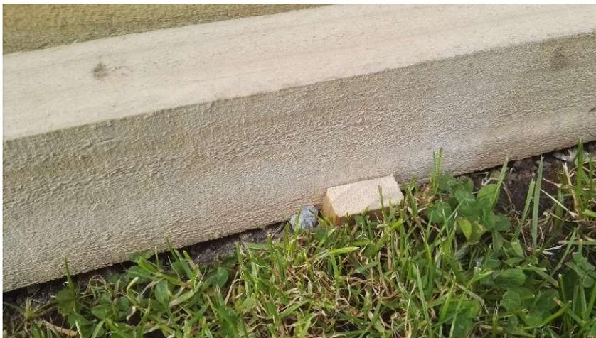
5. Fill inside the retaining board surround with base course up to about the 3/4 height of the surround. This will require about 900 litres of basecourse or one full trailer load. Compact using the bottom of the spade or by stomping on.
