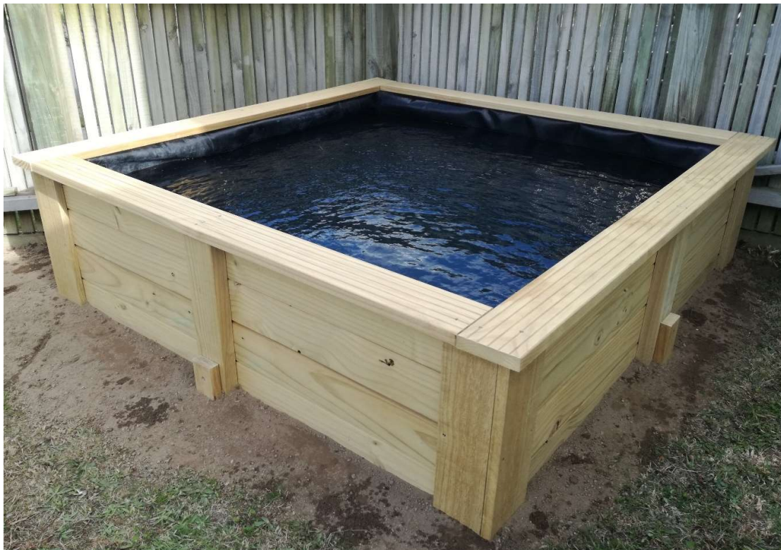
Fish pond built insitu with pond liner
