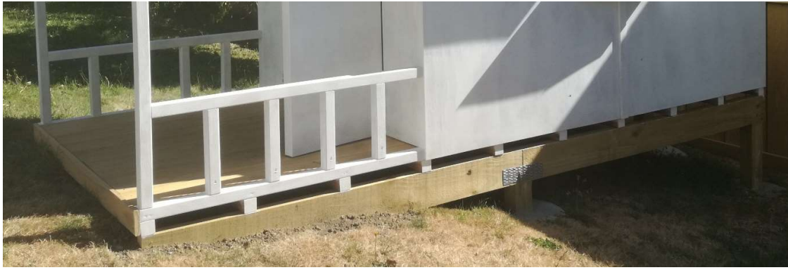
Elevated platform built to support wendy house on sloping lawn
