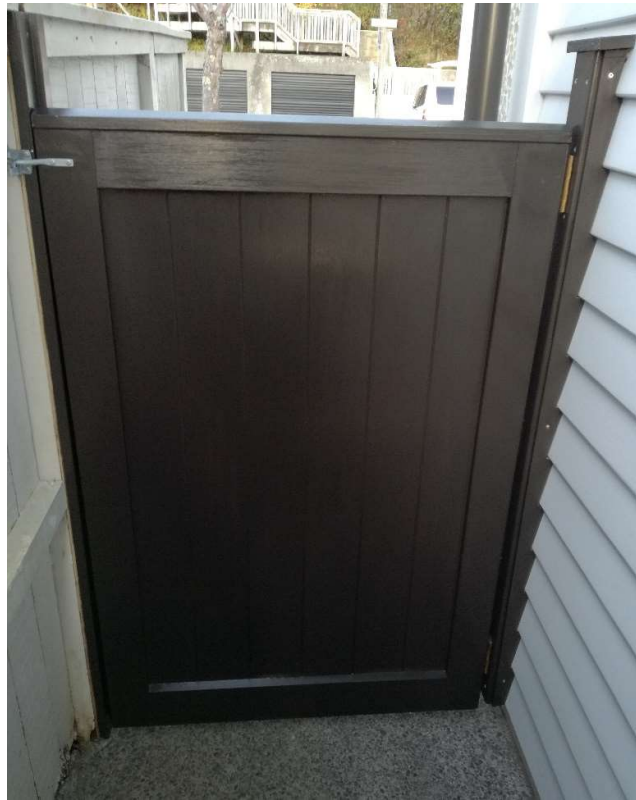
Painted tounge & groove pedestrian gate
