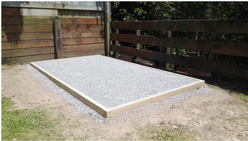
Raised plinth used to support floor of wendy house
