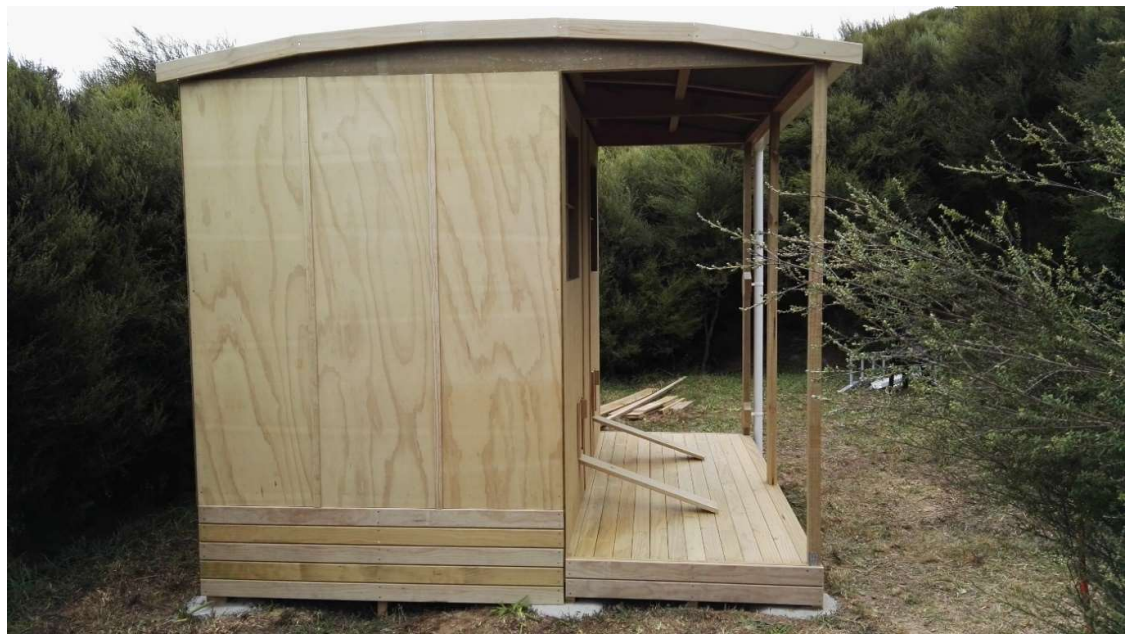
Chicken coop with curved roof profile built onsite
