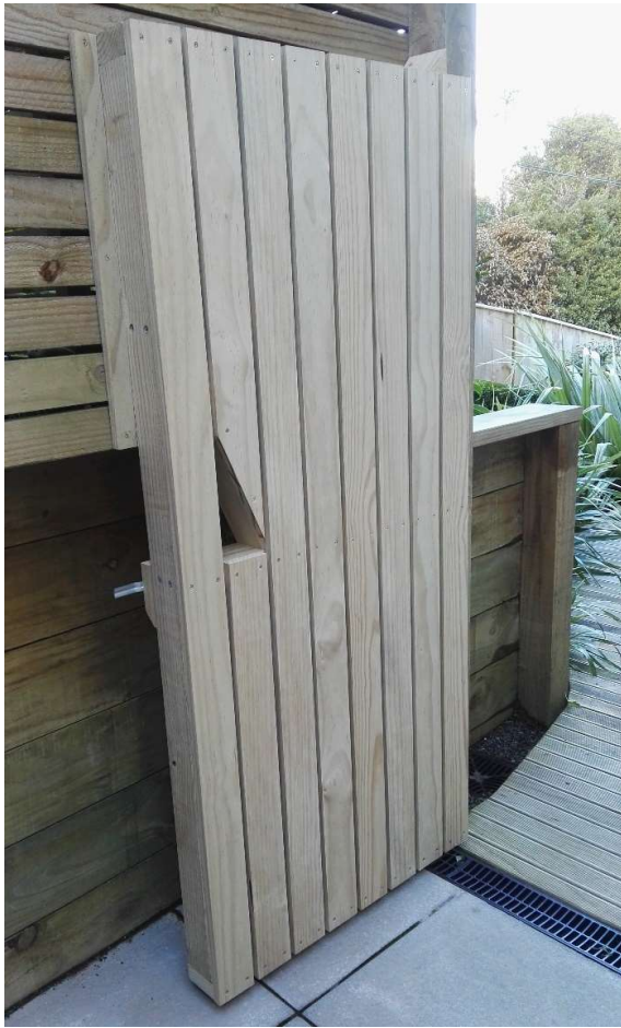
Pedestrian gate with vertical slats
