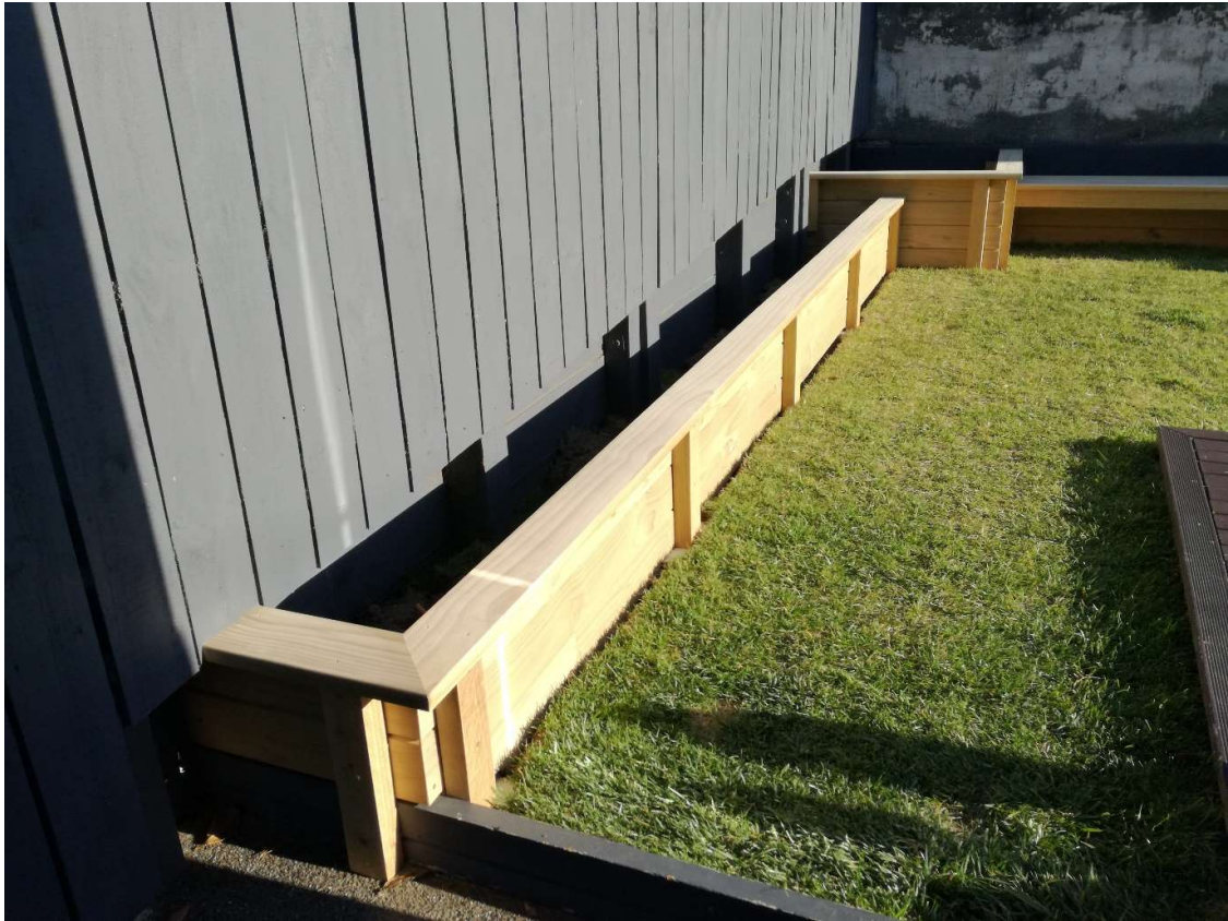
Planters built insitu against existing retaining wall
