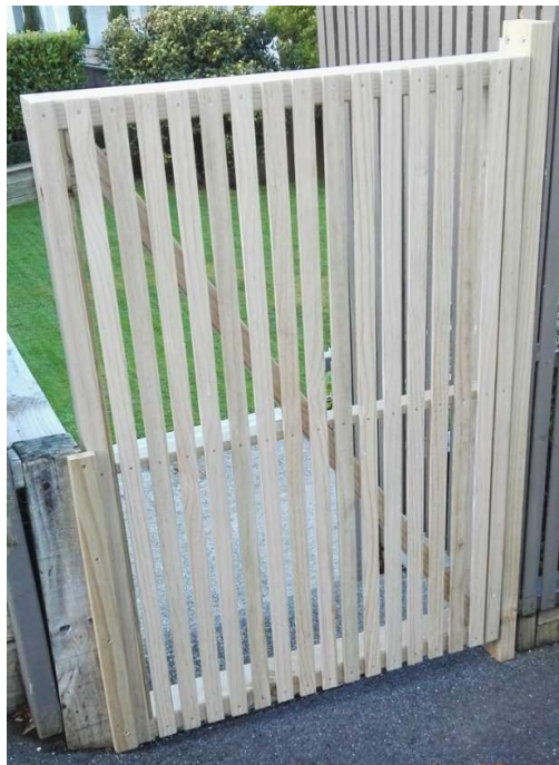
Pedestrian gate using trellis
