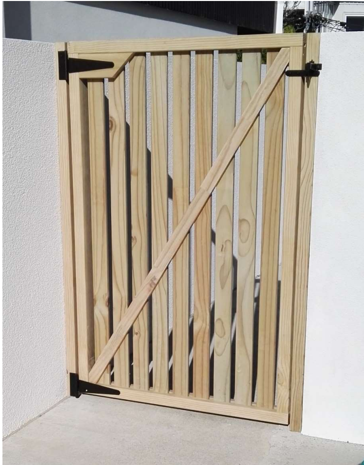
Pedestrian gate and jams secured to concrete block walls
