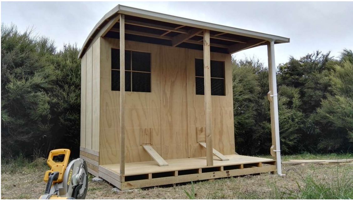
Chicken coop with curved roof profile built onsite
