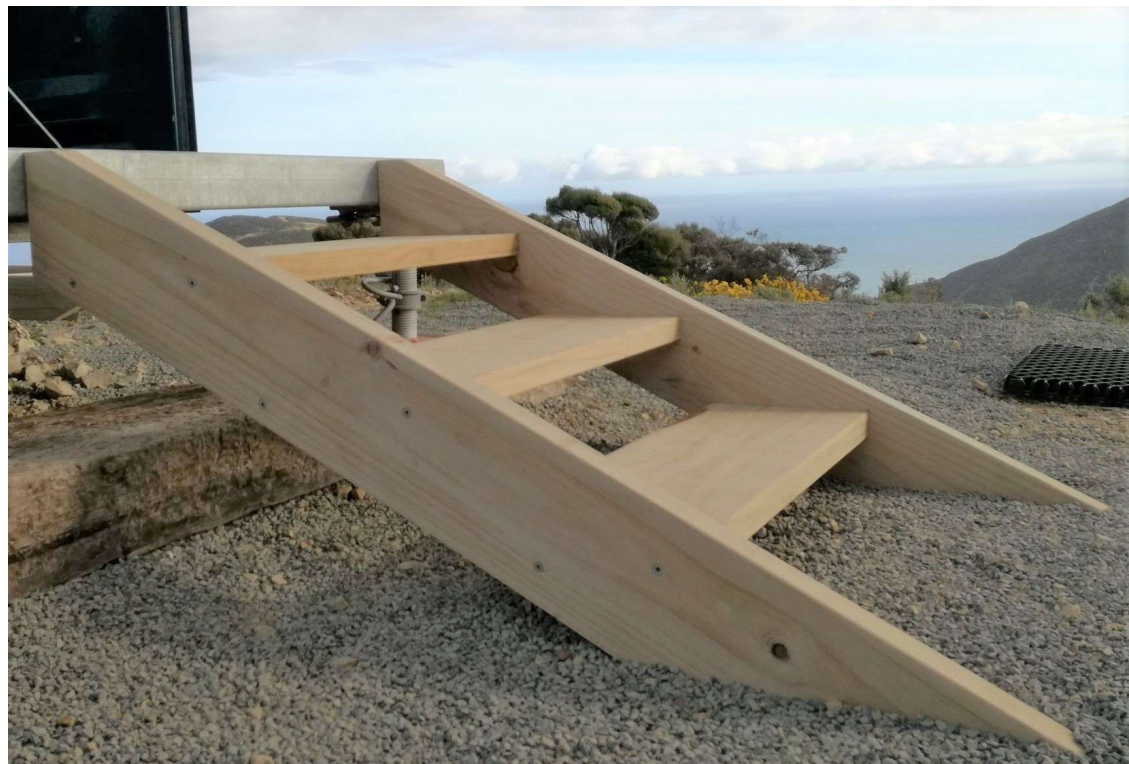
Custom fit pedestrian steps installed onsite
