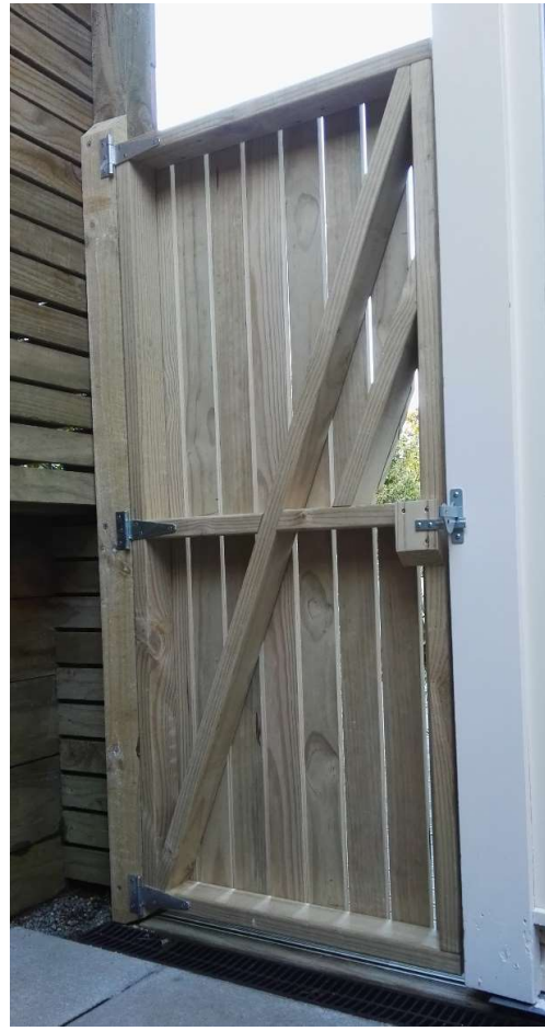
Pedestrian gate with vertical slats
