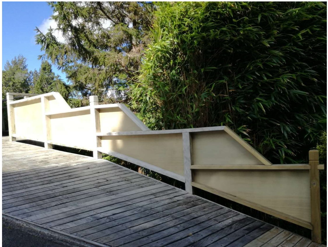
Fencing using plywood panels
