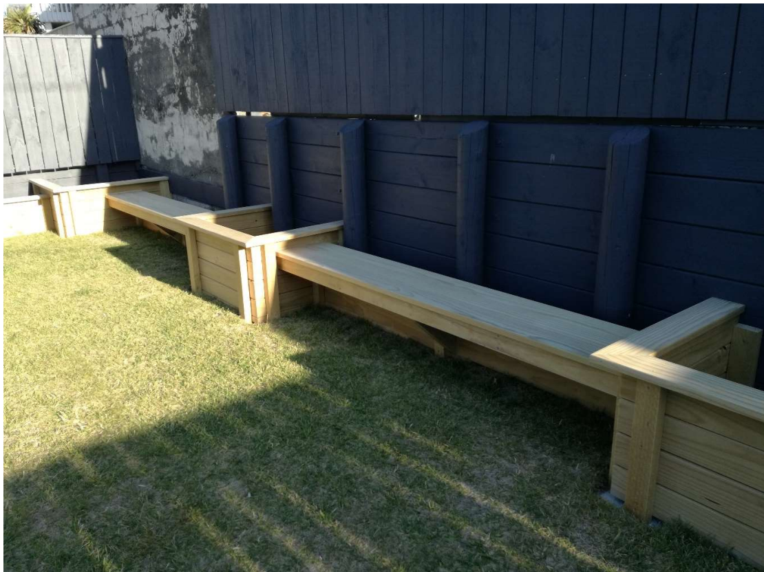
Planters and benchseats built insitu against existing retaining wall
