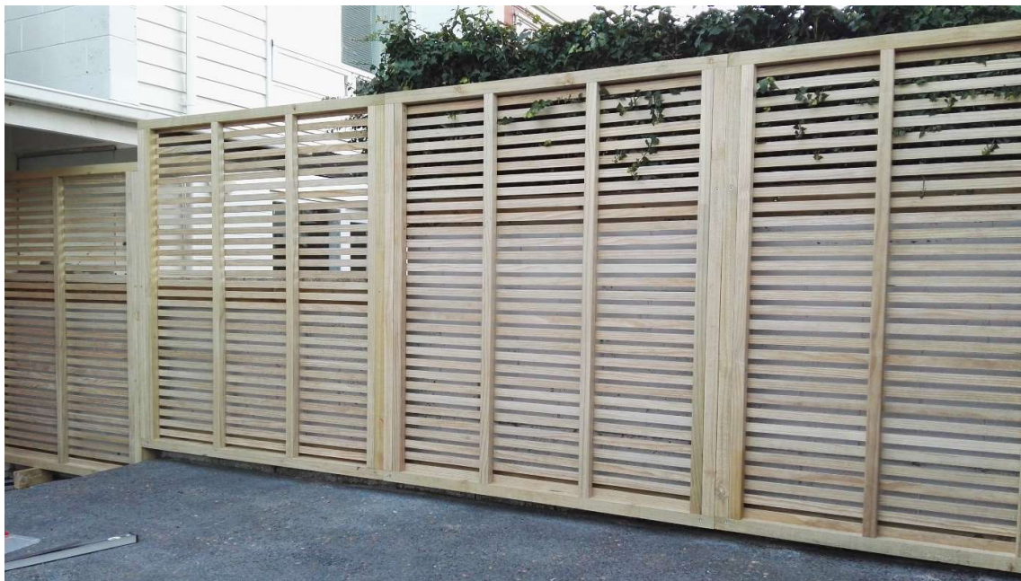
Trellis units attached together insitu to form screen fencing
