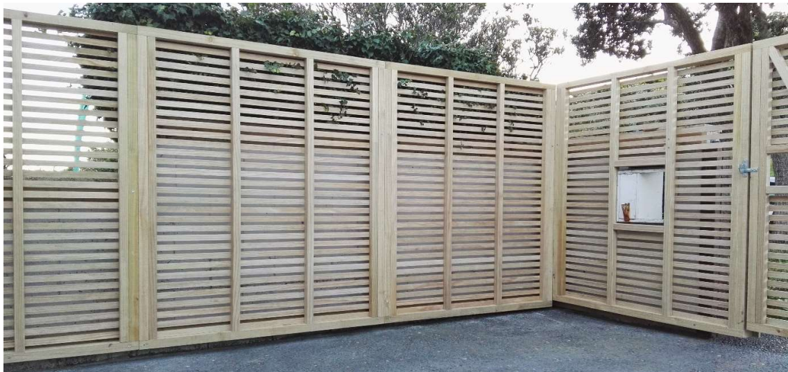
Trellis units attached together insitu to form screen fencing
